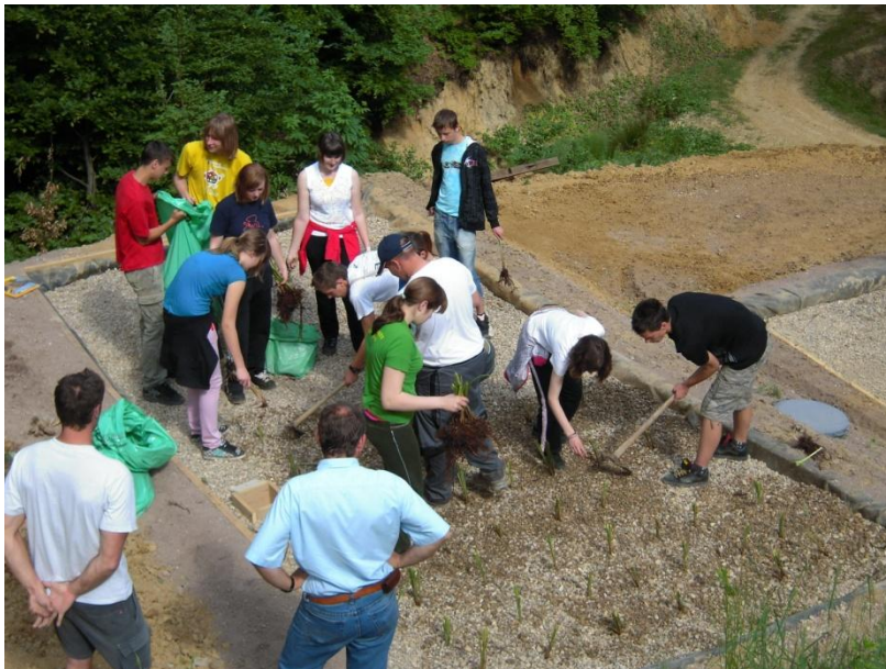
Picture 6. Planting Carex sp. on constructed wetland by students of nature conservation technician programme – ecoremediations.
